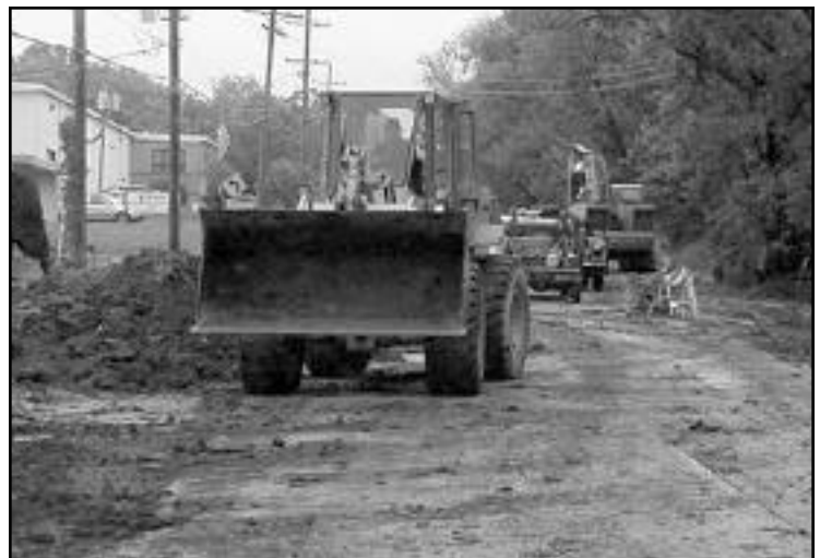
Crews work on reconstructing Lake Marian Road
