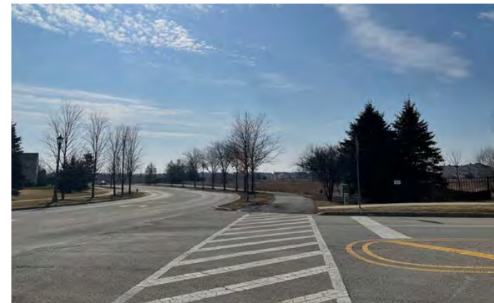
Sidewalk and pedestrian crosswalk improvements.
