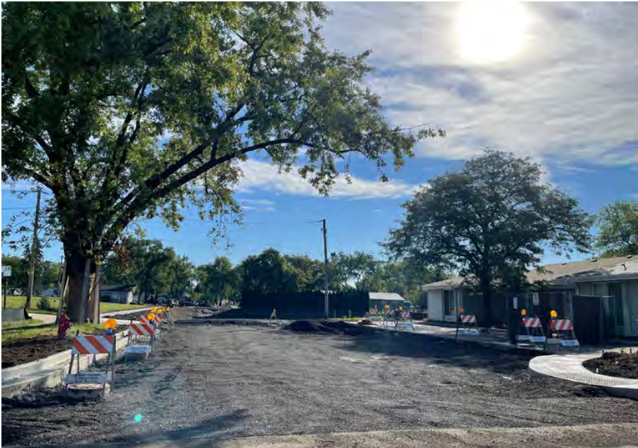
Road improvement in residential area
