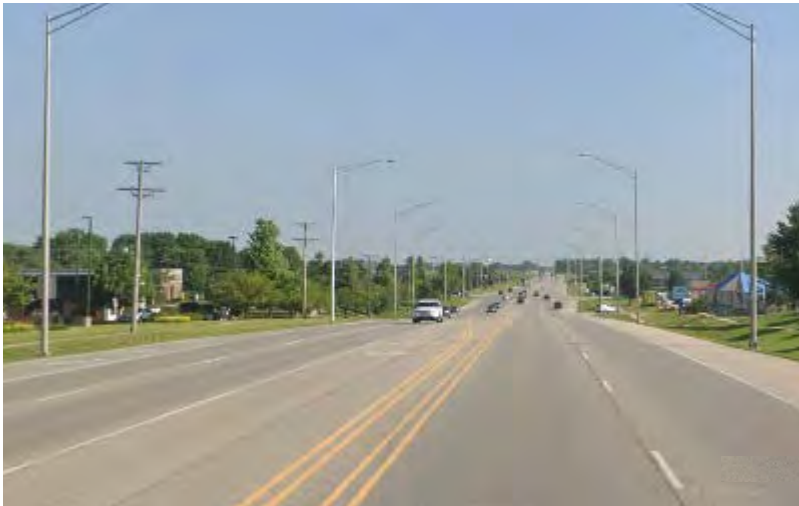
Randall Road going northbound.
